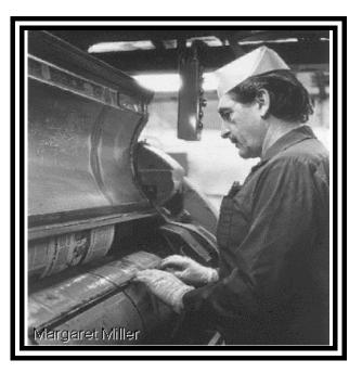
rolls of substrate. Presses that print on rolls, or webs, can achieve speeds of 600-900 m (2000-3000 ft) per minute. Presses that print on sheets are generally slower than web presses but can print on thicker substrates, such as Bristol board and sheet metal.
