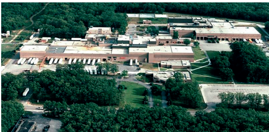
Sun Chemical's Muskegon, Michigan, USA pigments manufacturing facility
